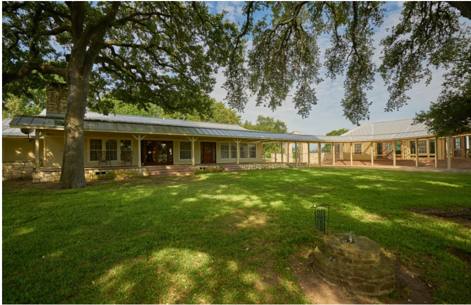
Back of House with Covered Walkway
