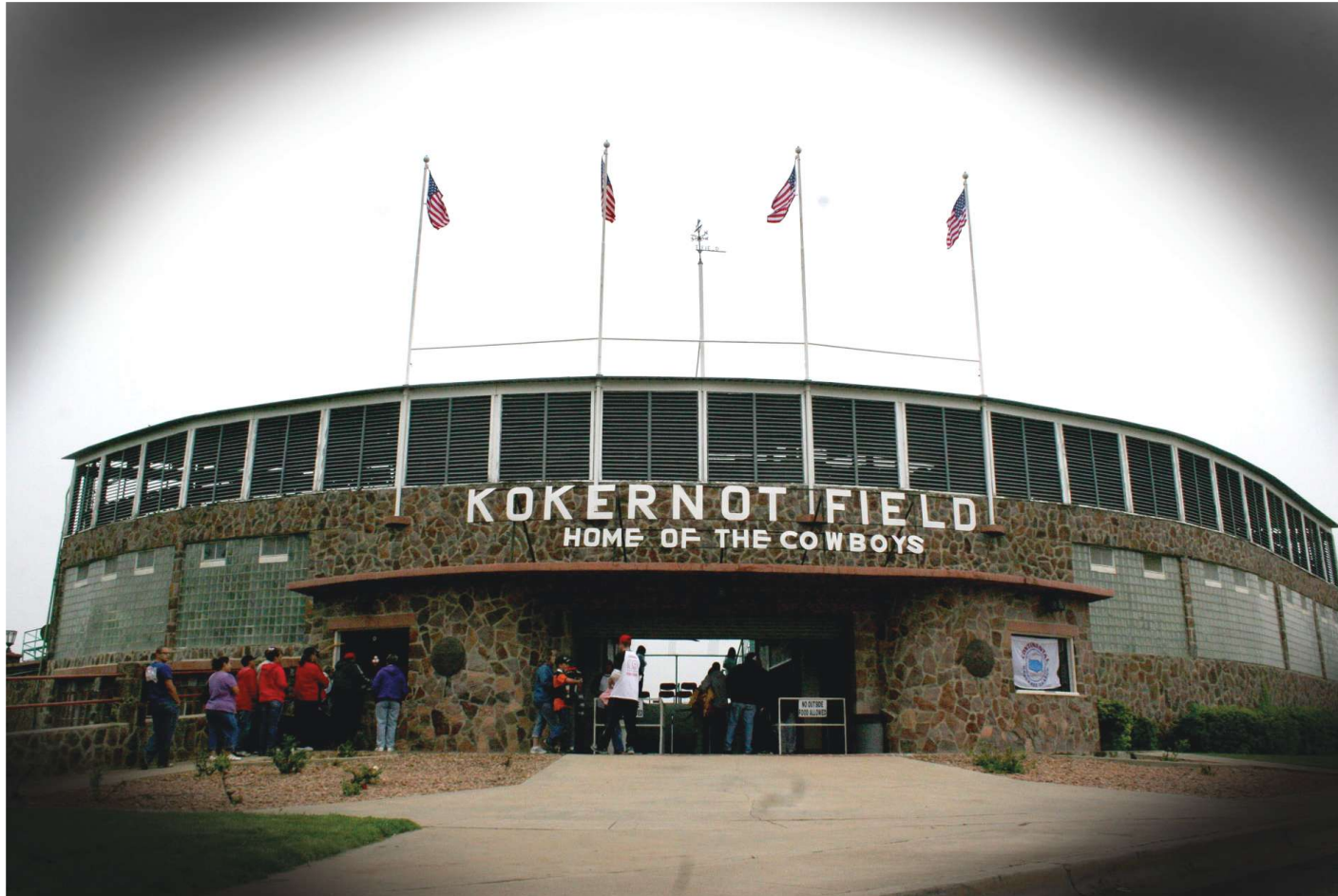
Christened “The Yankee Stadium of Texas” by Texas Monthly , Kokernot Field (above) was built in 1947 by H.L. “Mr. Herbert” Kokernot Jr. The family’s o6 brand is evident throughout the ballpark.
